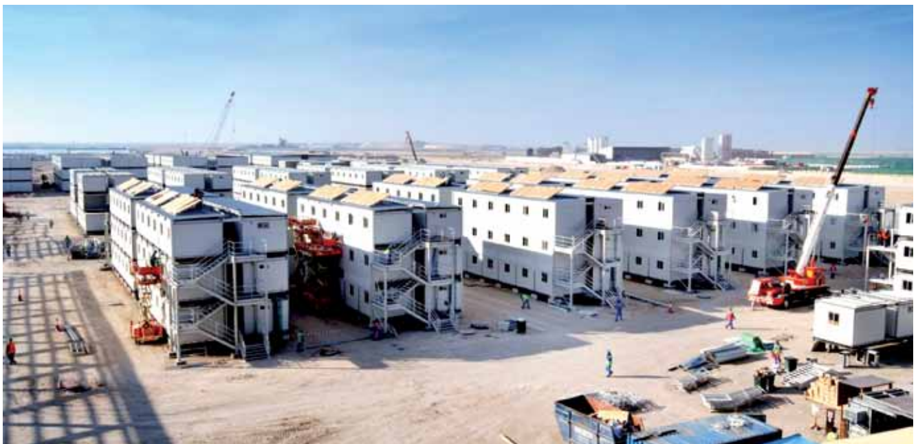
Saadiyat Construction Village ▼ Abu Dhabi
