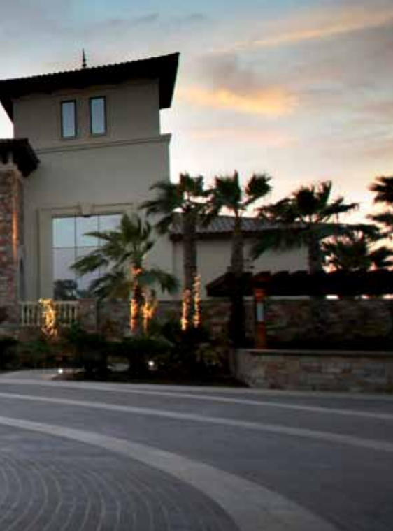
Saadiyat Beach Golf Course ▲ Academy building main entrance
